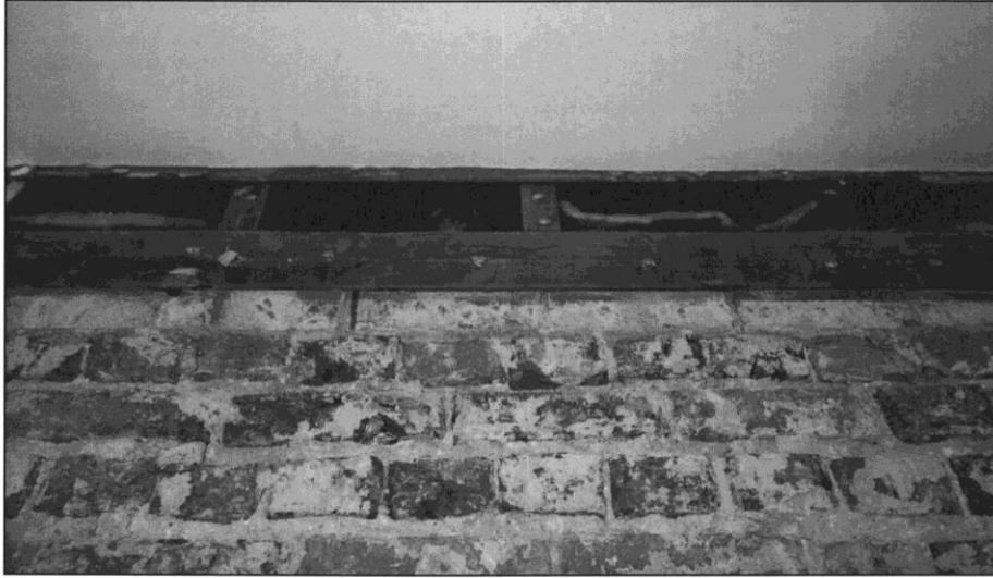
Figure 17: Modern brickwork to top of wall
