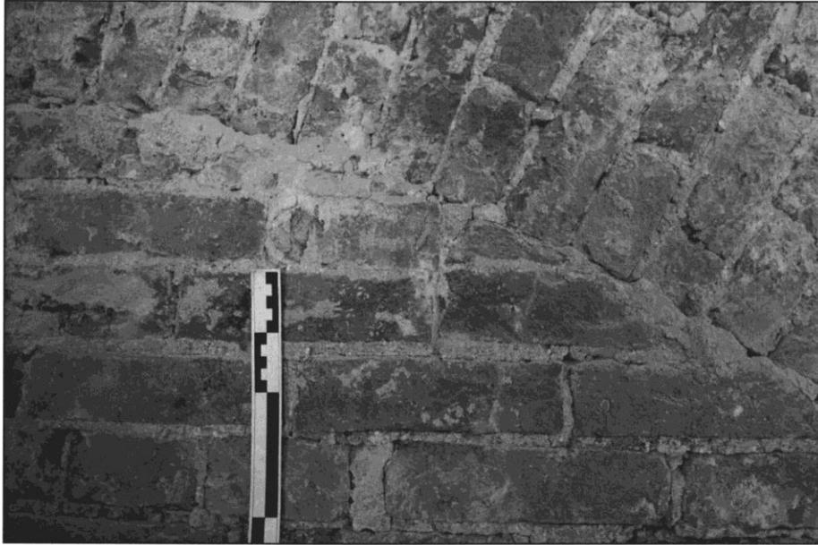
Figure 14: Size of bricks and mortar to infilled archway with scale
