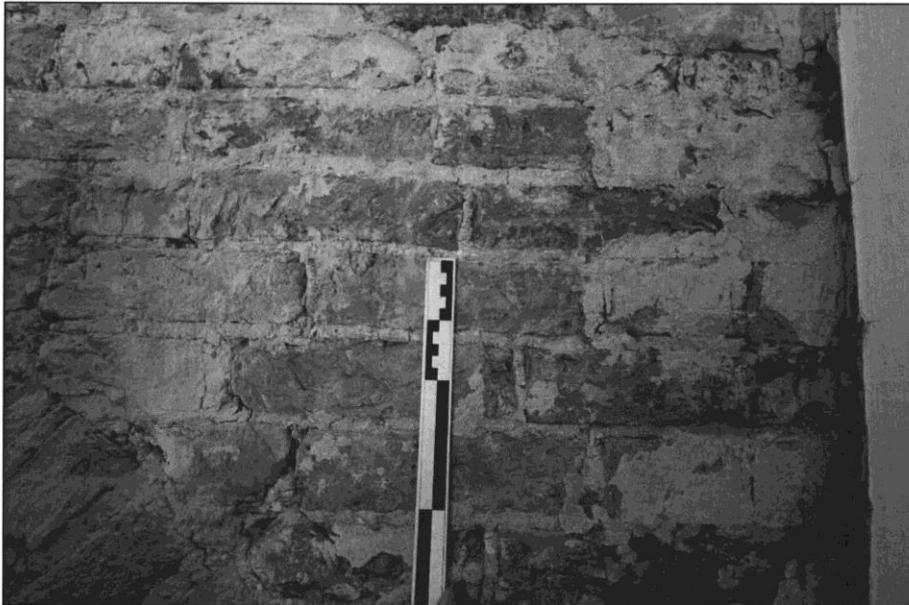
Figure 13: Size of bricks and mortar to main body of wall with scale
