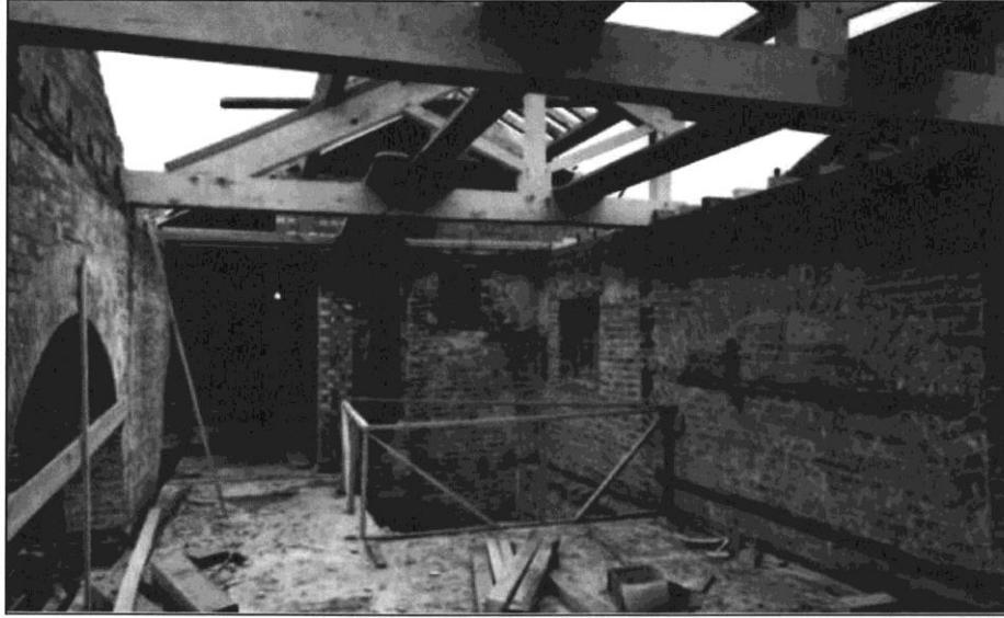
*Figure 11: Photograph from 1970s works showing the infilled arch on the eastern elevation (arch to east on right hand side)*
