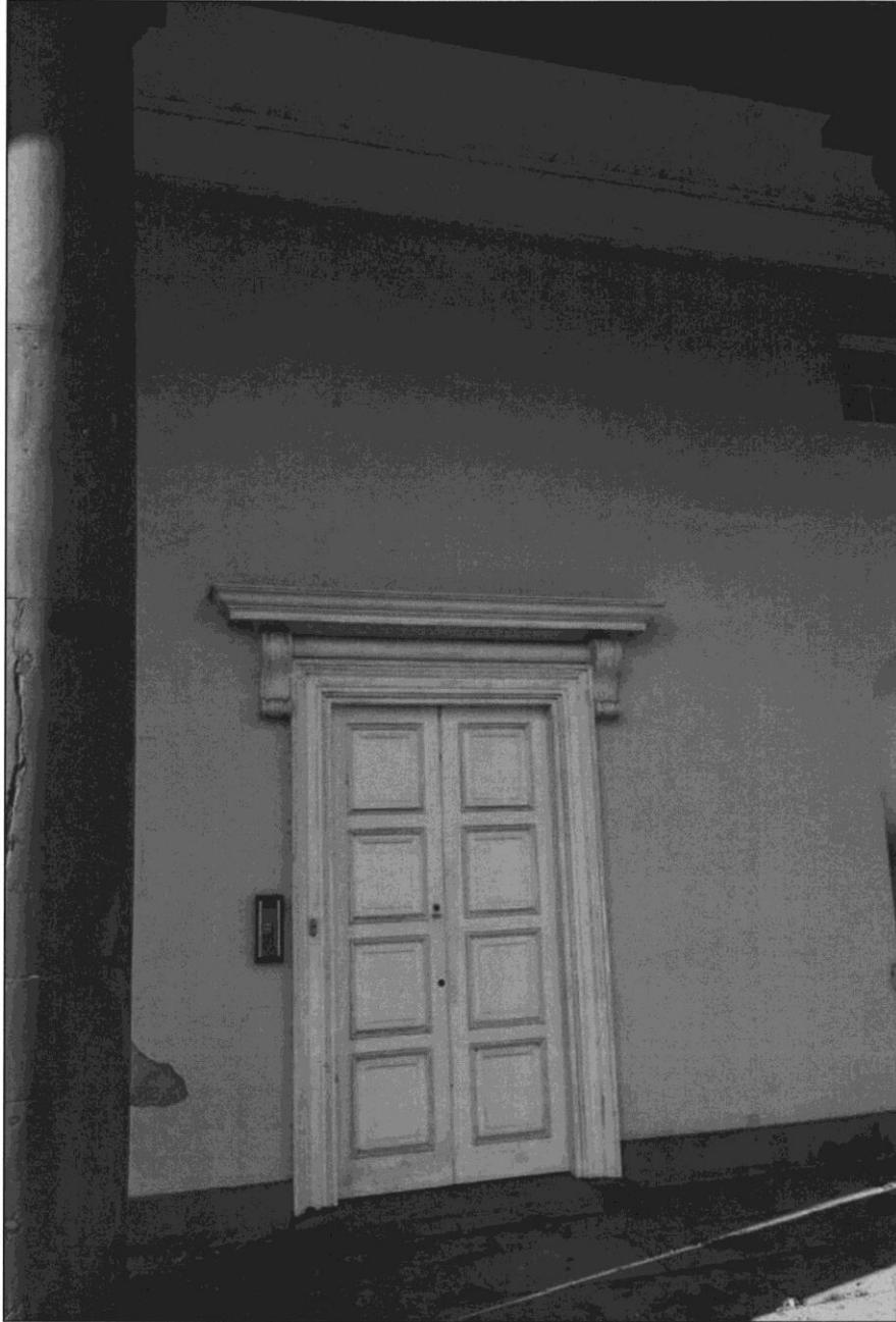
*Figure 12: Ghost archway visible on external eastern elevation above door*
