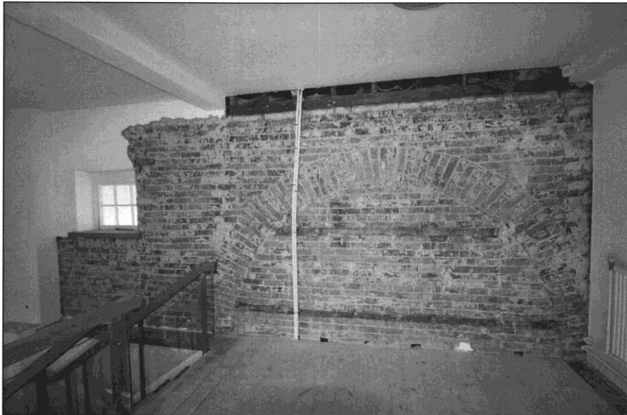
Figure 15: Slightly darker bricks to the left hand side of photograph in the main wall compared to infilled archway
