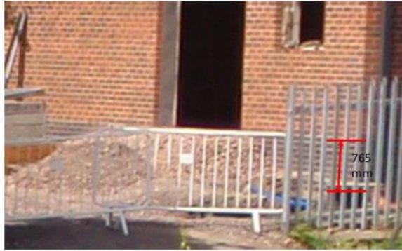
From original ground level to top of blue bricks is approximately 9 bricks at 75mm height. Allowing for a 10mm bed gives 765mm
