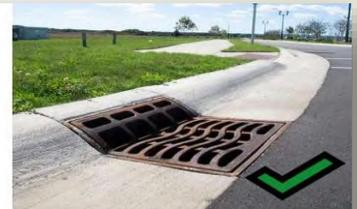
combination 'well' and kerb drain, set into concrete roadside edging
