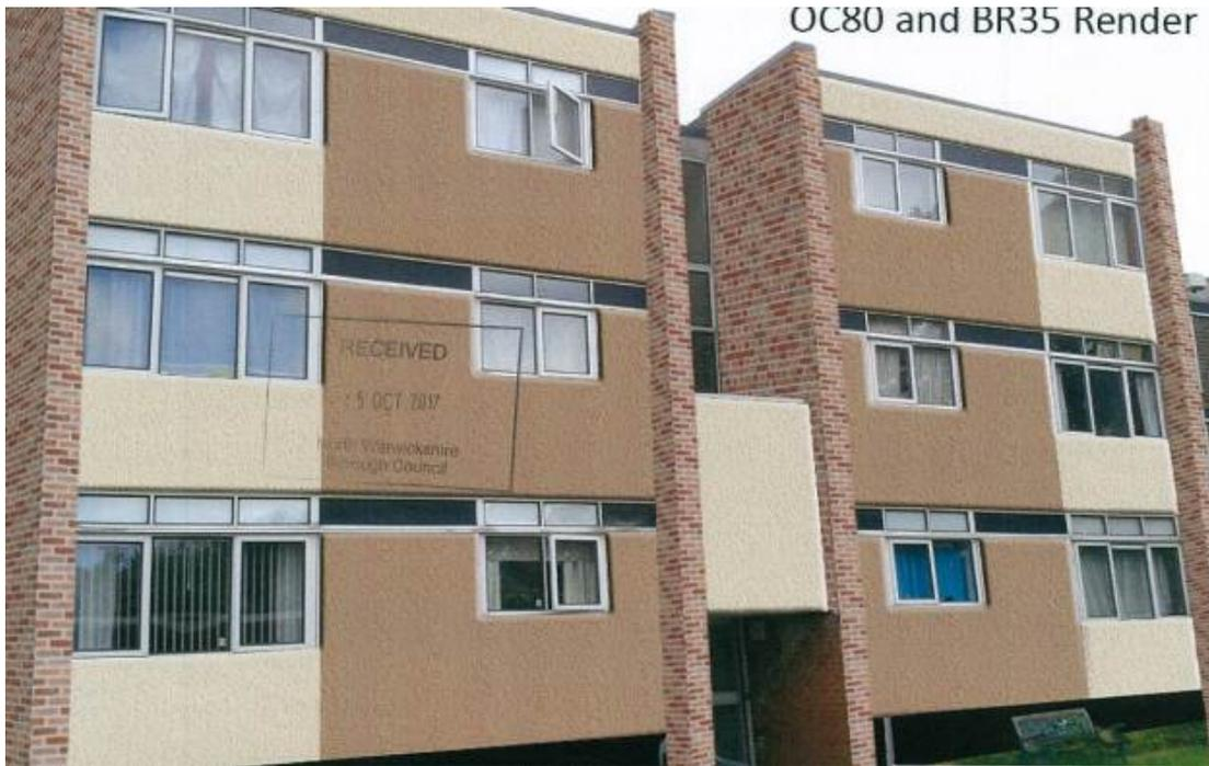
***Proposed rear elevation with a contrast light cream and mid brown rendered effect external wall insulation***
