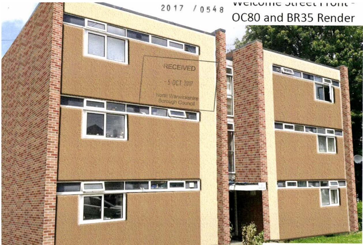
***Proposed front elevation in contrast cream and mid brown render effect external wall insulation***
